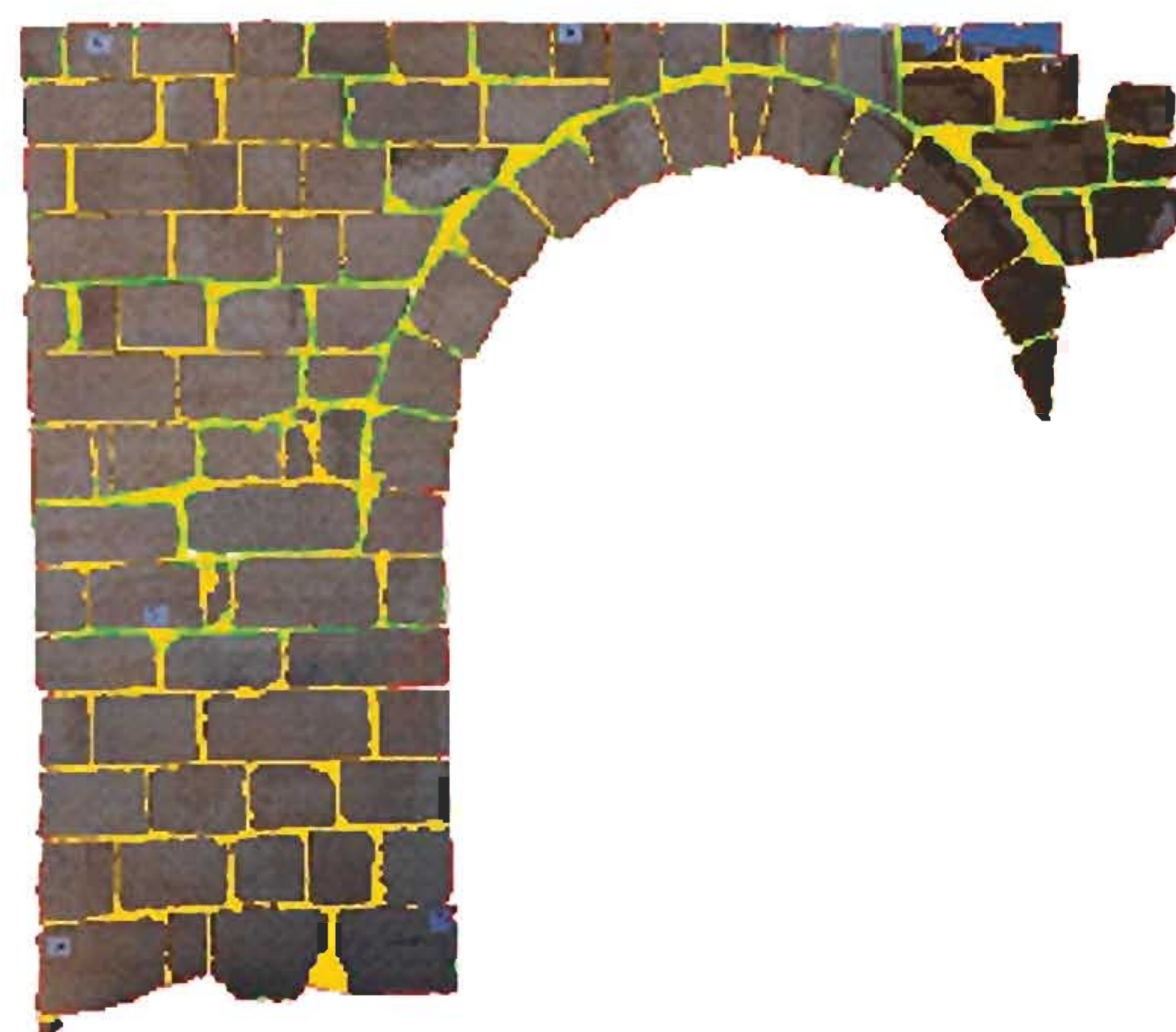
Fig. 12 Orthophoto generation on a query related to blocs, with design of USM perimeter and the cement paint in yellow
