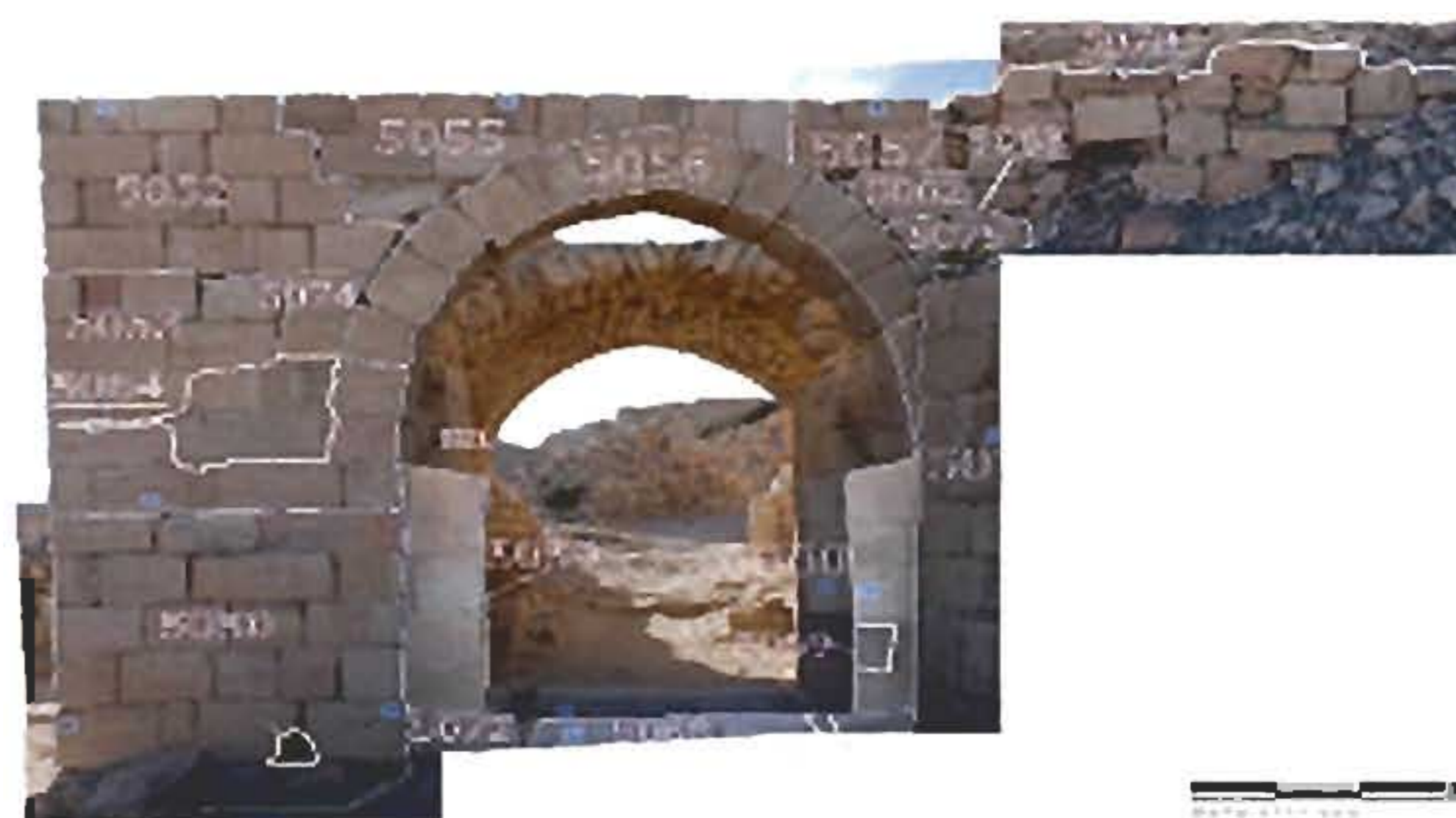
Fig. 10 Orthophoto with manual design of USM.
