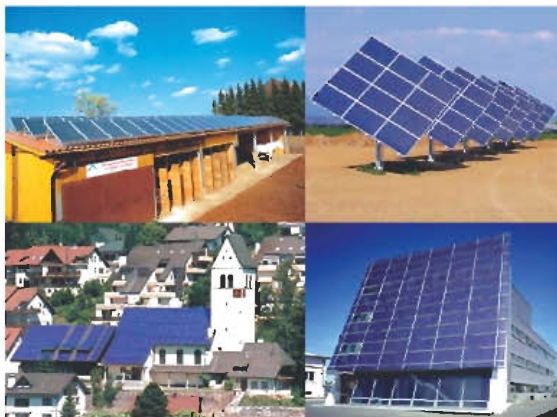
Fig. 2 Ground-mounted and building-integrated photo-voltaic arrays.
