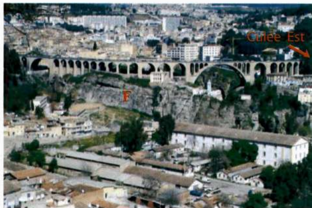
Photo 1 - Le pont de Sidi Rached à Constantine Sidi Rached bridge in Constantine
