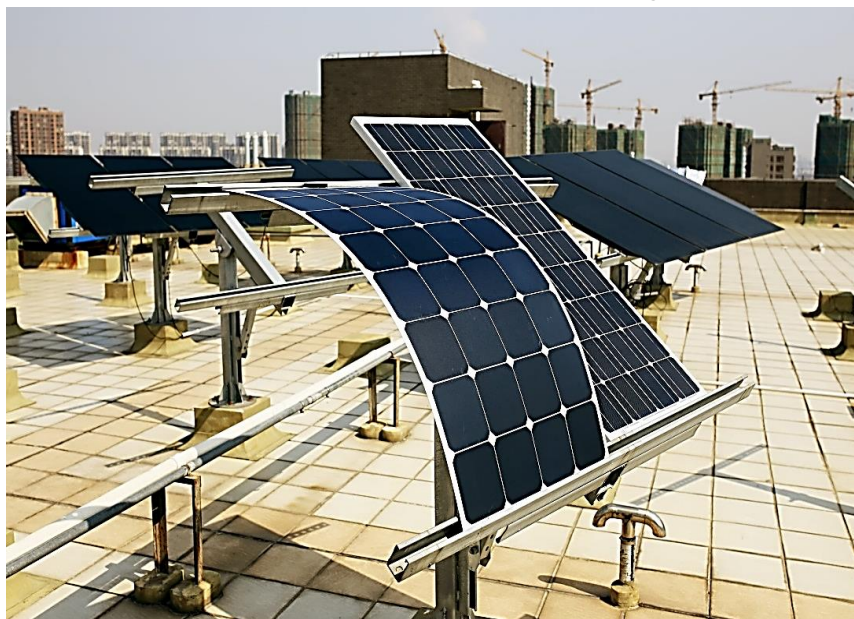
Figure N°02: Thin-Film Solar Panel (left) and Rigid Solar Panel (right)
