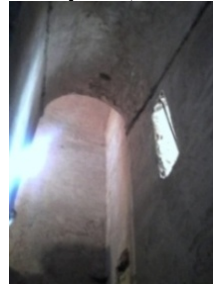
Fig.50: berceaux rampants, M6
