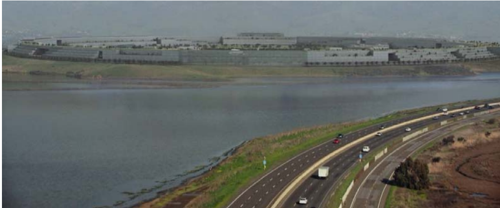
Fig. 1. The Circle, the building as a utopia
