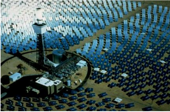
Fig.2: Heliostats solar power tower field [2]
