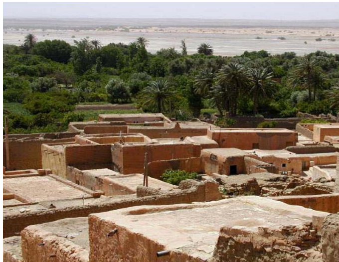
Fig. 1: Roofs exposed to solar radiations
