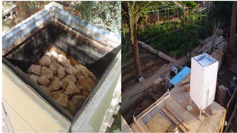
Fig. 4: The evapo- reflective roof
