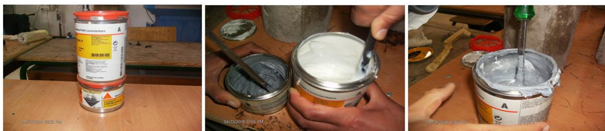
Fig 2. Preparation of resin (Sika Dur 330).
