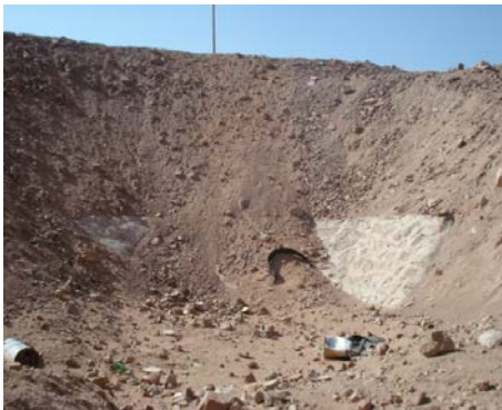
Fig. 20. The lack of protect culvert from soil erosion
