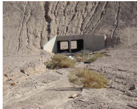
Fig. 20. The lack of protect culvert from soil erosion
