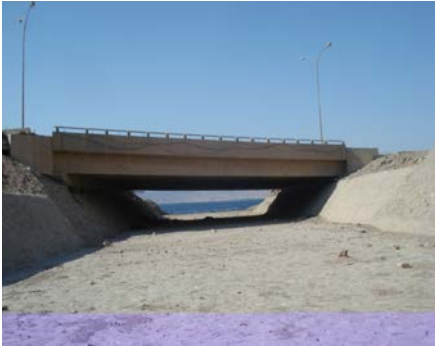
Fig. 18. Bridge before the flood
