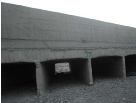
Fig. 16. Culvert before the flood
