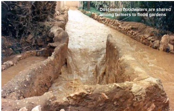
Figure 24: A seguia carrying water from a flood toward the various gardens for temporary flooding (Photo M'zab Valley Archives)
