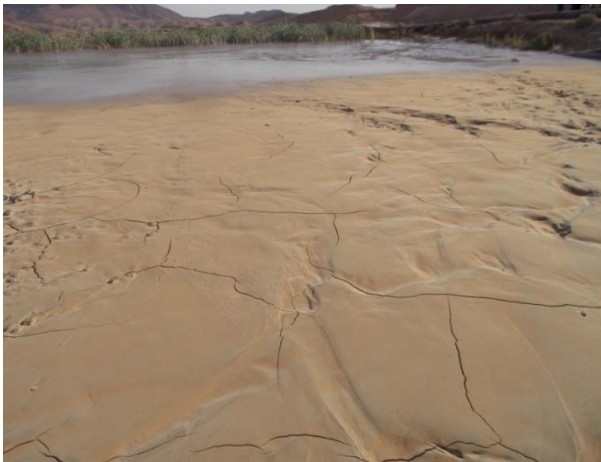
Figure 8: Basin filled with silt spilled during dredging of the Foug El Gherza dam reservoir (Photo. Remini 2017)
