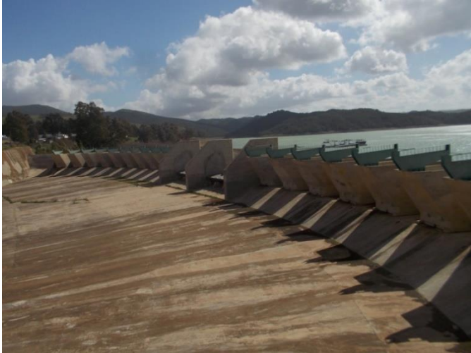
Figure 11: The Ghrif dam spillway equipped with fusegates (Photo. Remini, 2018)
