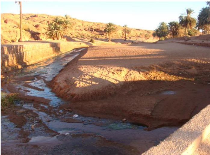
f) Dam after the passage of the 2018 flood-The silt is more important than before the desilting. View from upstream (Photo. Remini, 2018)
