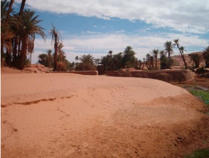
a) Dam before the 2017-Silted Reservoir (Photo. Remini 2008)
