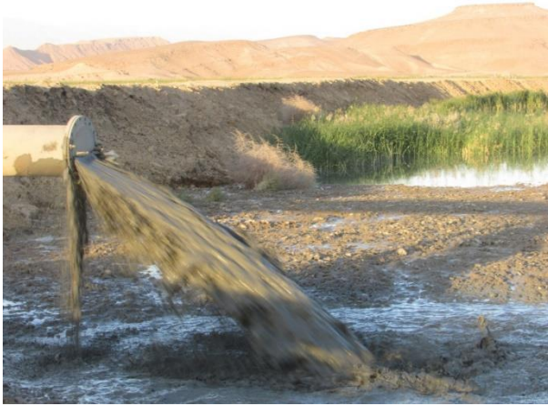
b) Dredging operation carried out on the Foum El Gherza dam reservoir in 2017 (Photo. Remini, 2017)
