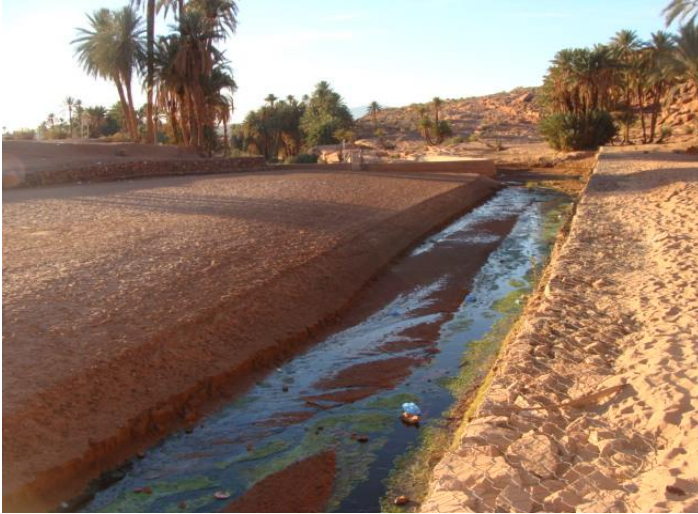
e) Dam after the passage of the 2018 flood-The silt is more important than before the desilting. The dike is hidden by mud (Photo. Remini, 2018)
