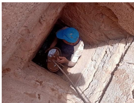
b) Cleaning of vertical shafts
