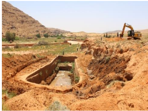
a) Rehabilitation of the source “Tafssast”
