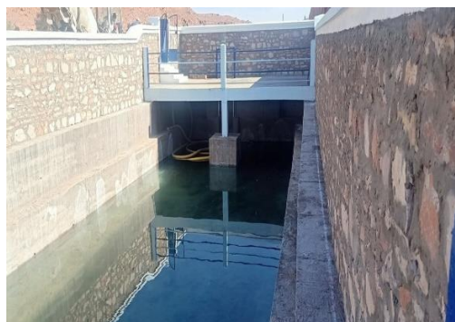
Figure 8. Tafssast Spring after rehabilitation works (Derdour, 2021)
