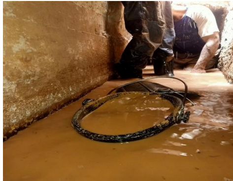
c) Cleaning of underground canal (Tissfalt)
