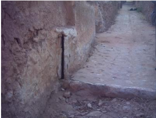
Figure 29: A Koua with the Rosfa in an alley of the palm grove-East from Ghardaia (Photo. Remini, 2006)
