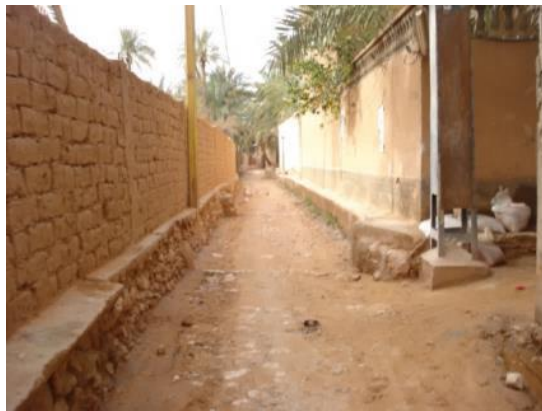
Figure 25: Segua with a frontal elevation for the circulation of the population in period of flood (Photo. Remini, 2013)
