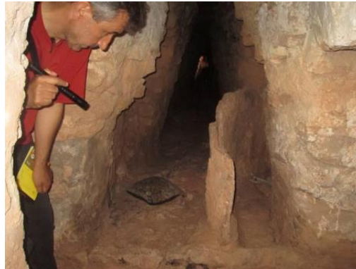
Figure 16: A distribution point of the waters inside the Galleries (Tissanbadh N'Bouchemdjane) (photo. Remini, 2013)
