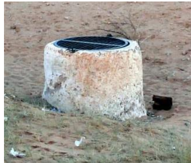
Figure 15: Galleries ventilation well (Tissanbadh N'Bouchemdjane) which can reach 40 m deep (photo. Remini, 2010)
