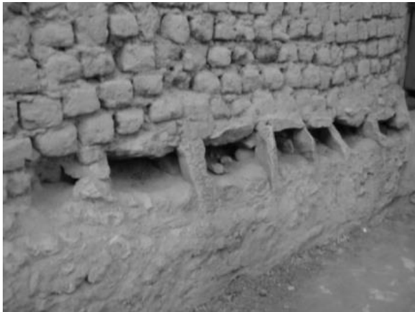
Figure 31: A system for discharging flood water from a garden in the palm grove of Ghardaia (Photo. Remini, 2013)
