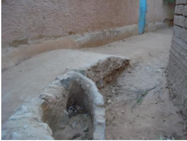
Figure 30: A donkey shaped obstacle to direct the flow without disturbing the circulation of the population (Photo. Remini, 2010)
