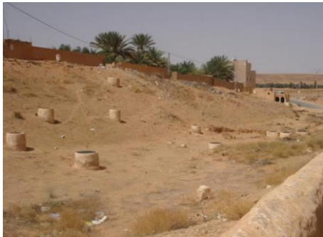
Figure 14: A view of the ventilation shafts of the galleries (Tissanbadh N'Bouchemdjane) in Ghardaïa (photo. Remini, 2010)
