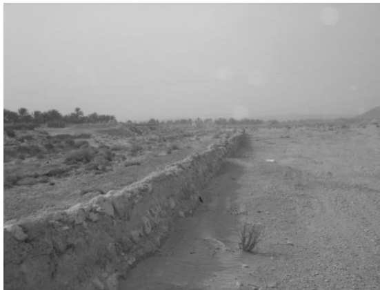
Figure 6: The wall dividing the M'zab River into three seguias (Photo. Remini, 2014)
