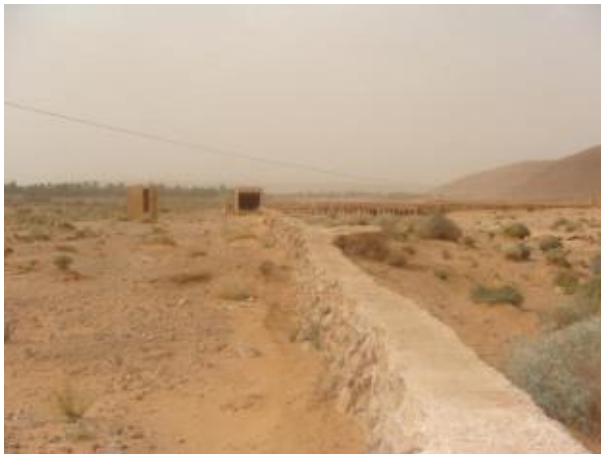
Figure 7: A view of part of the rock wall (Photo. Remini, 2010)
