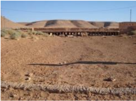
a) Upstream view
