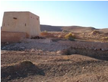
Figure 25: Second Dam - Part of the spillway (Photo. Remini, 2013)
