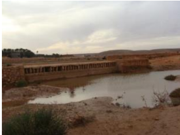
Figure 44: Spillway from the Bouchen dam (Photo. Remini, 2013)
