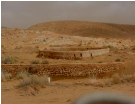
a) Diversion structure
